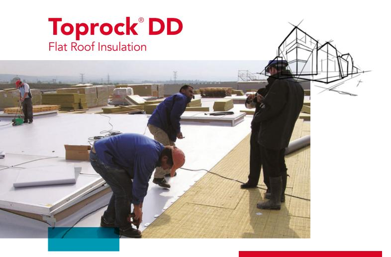
ROCKWOOL TOPROCK® DD is a high-density, uncoated stone wool insulation board for low-slope roof applications. TOPROCK® DD is a suitable substrate board for all low-slope roof decks and is compatible as the substrate for mechanically attached membrane systems.
